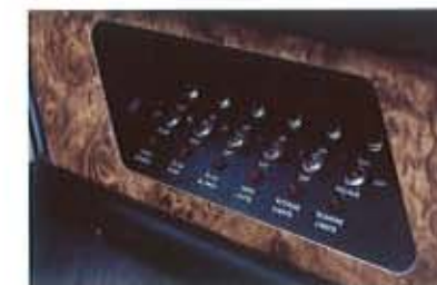
Electrical circuits are protected by circuit breakers.
