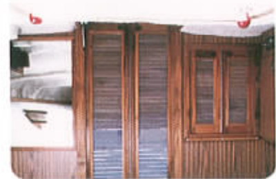
Louvered teak doors are fitted with insect screen on the cabin side.
